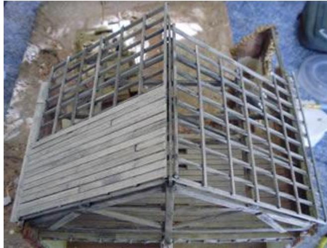
We have now stuck down the roof battens. If this was a clay tiled roof they would be smaller and closer together so the clay tiles could hang from them. We have started to cover the battens with planks which intern will be covered with slate roof tiles. Slate tiles can also be attached straight onto the battens. It all depends on the building you are modelling.
