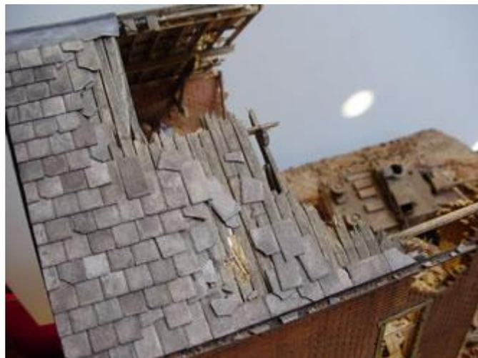
**Note:** *The first row of slate tiles are laid long ways running parallel with the roof (you can see this at the bottom right of the roof in the picture above). The second row completely covers the first. The gaps in second row should not be directly above the gaps in the first row.*
