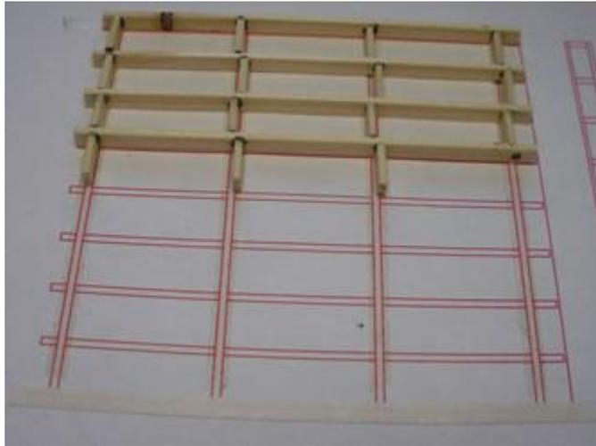
Attach double sided tape to the drawing to hold down the wooden floor joists and noggings.
