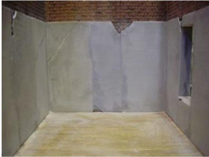
Use the diluted filler to fill the gaps between the plaster sheets. Paint it on then scrap off the excess with a straight edge. Once dry you can give it a light sand and paint or wall paper the walls.
