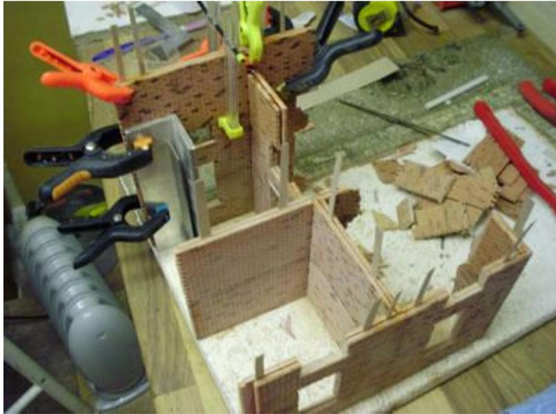
We clamped some aluminium angle to the wall to keep the next layer of walls section vertical and flush.
